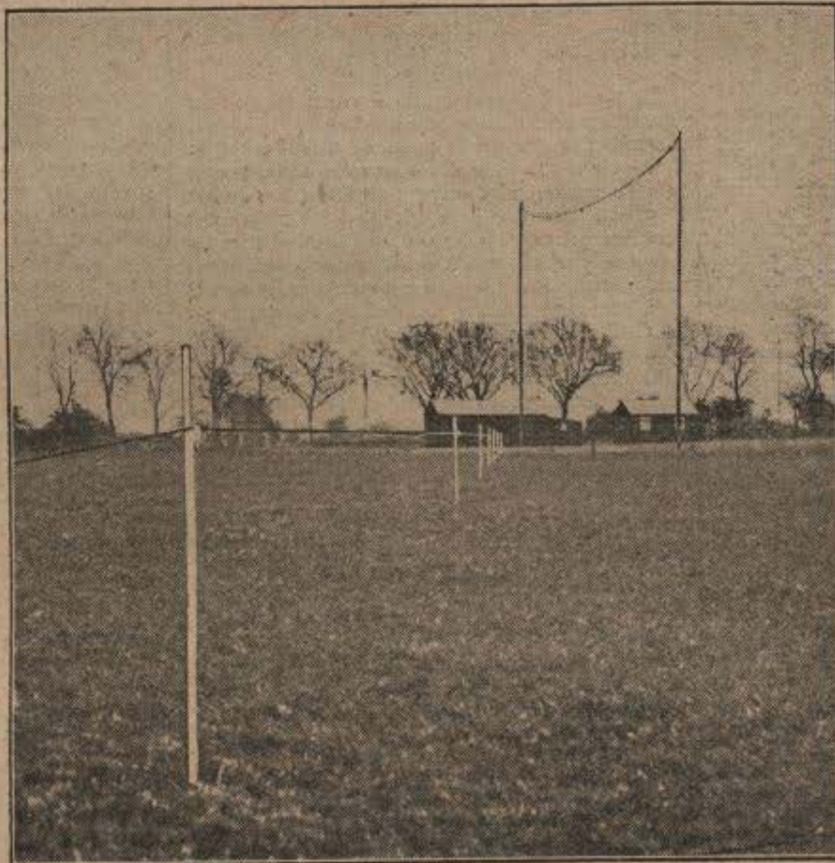
B.B.C.'S RECEIVING STATION AT KESTON.
